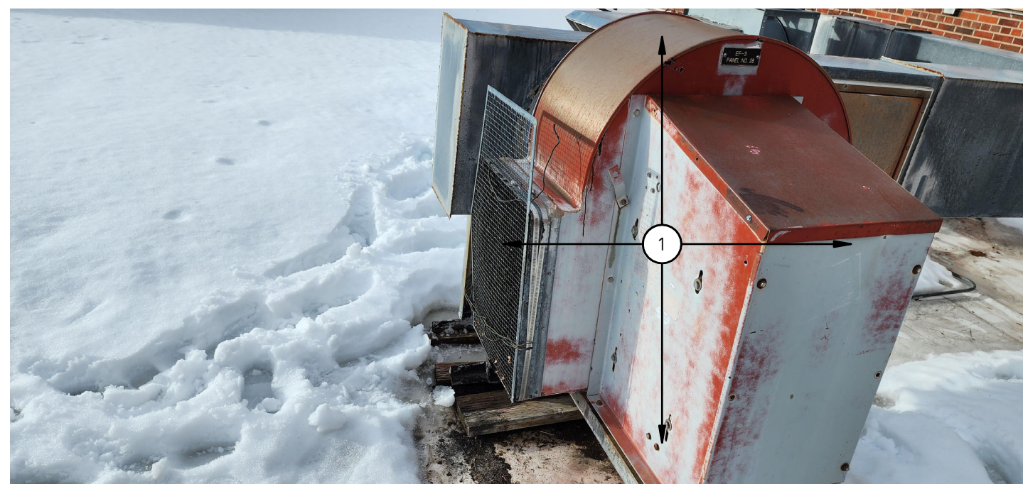
5 ROOF PHOTO A4.1 NOT TO SCALE
