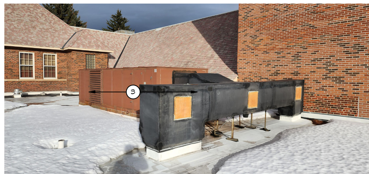
7 ROOF PHOTO A4.1 NOT TO SCALE
