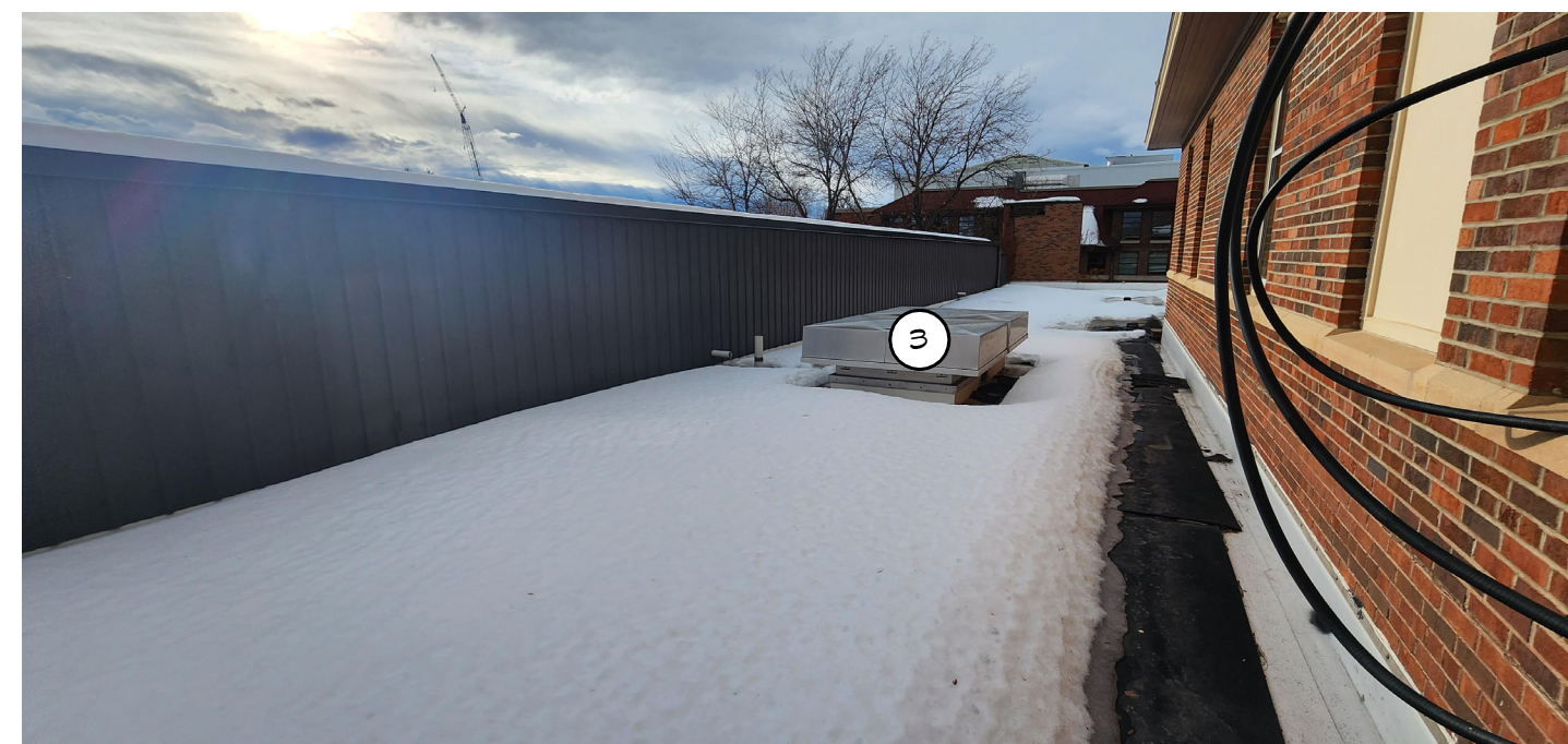
6 ROOF PHOTO A4.1 NOT TO SCALE
