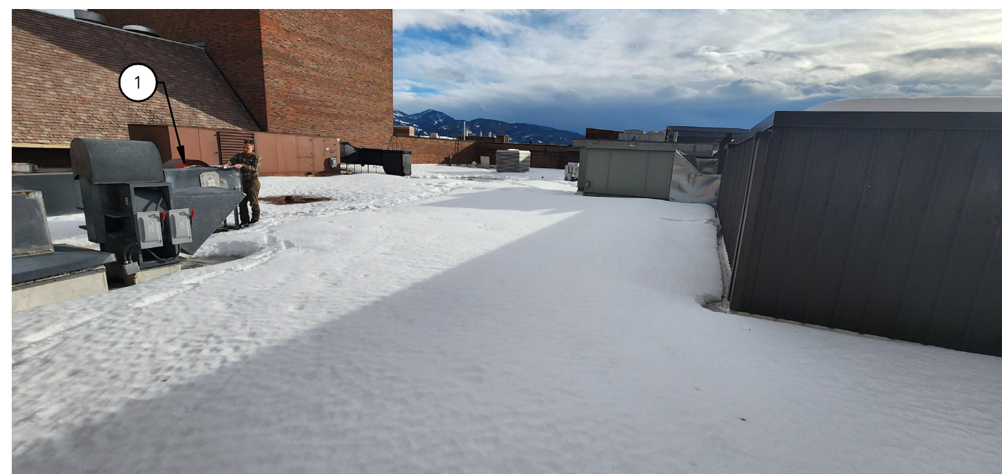
3 ROOF PHOTO A4.1 NOT TO SCALE
