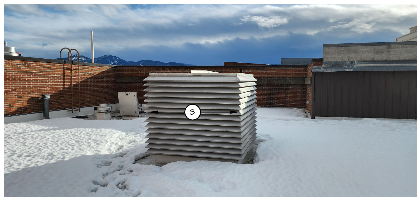
8 ROOF PHOTO A4.1 NOT TO SCALE
